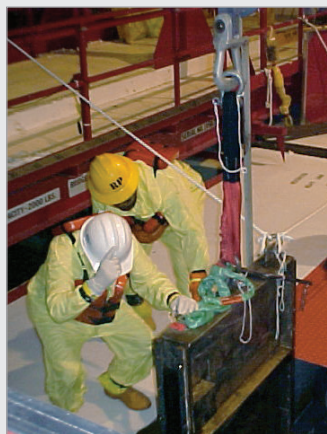
Spent Fuel Pool Gate - Install
