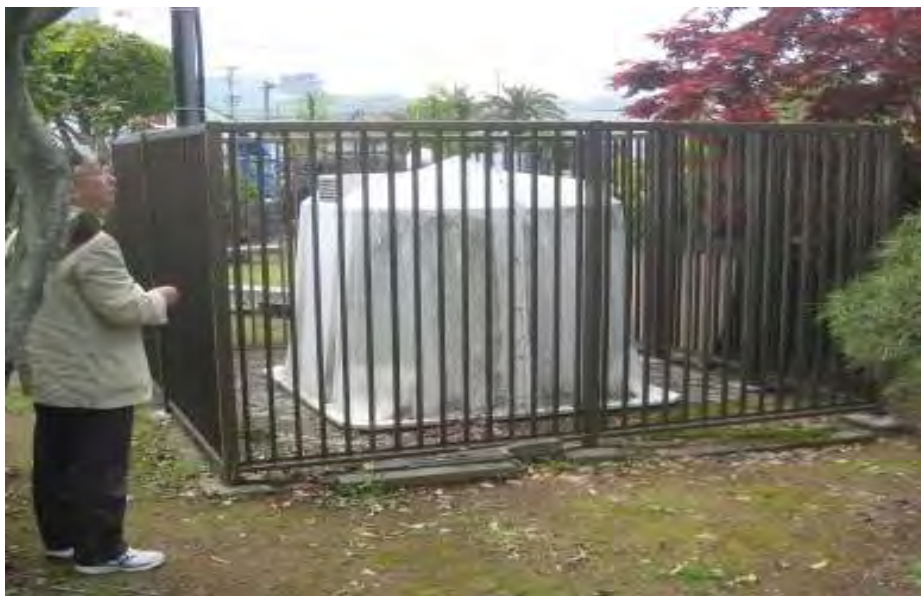
The most serious damage in the Uto area was partial collapse of the city hall due to failure in the main concrete columns. The Uto strong motion recorder is housed in a small enclosure on the city hall grounds (lower photo).
