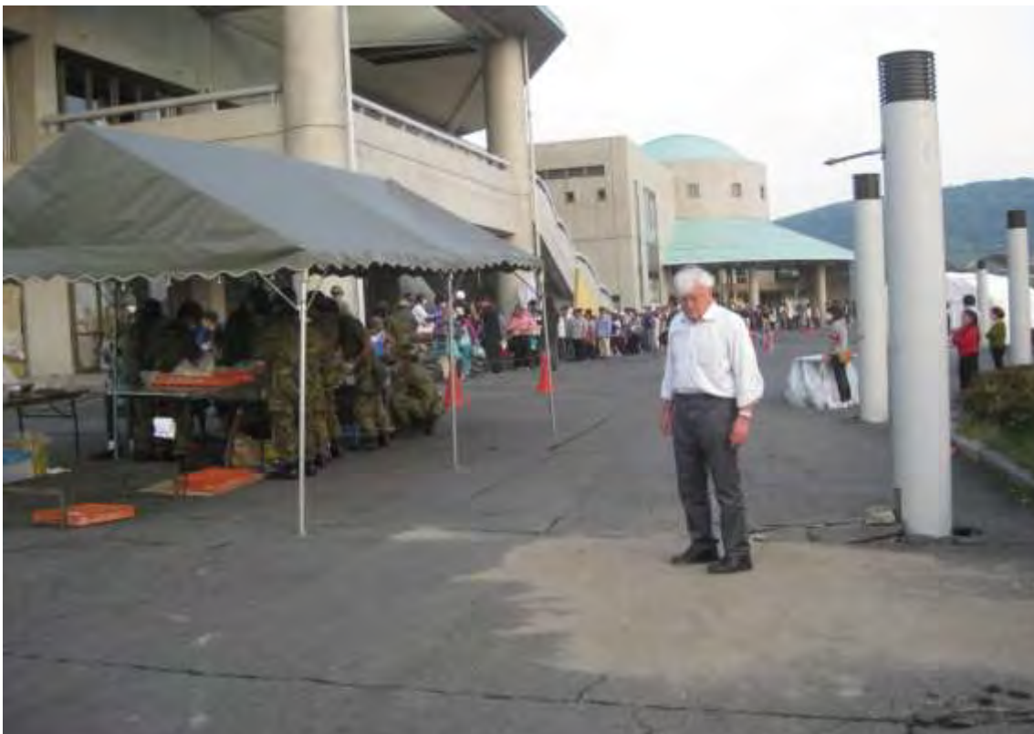
The Mashiki sports complex is a two-storey concrete shear wall structure designated as the emergency shelter and supply distribution point for the most heavily damaged area. The soft soil at the center of the valley displayed severe settlement, creating permanent waves and offsets in the pavement where the local population lined up for supplies. Pockets of liquefaction were indicated by sand boils as shown at lower right in the lower photo.
