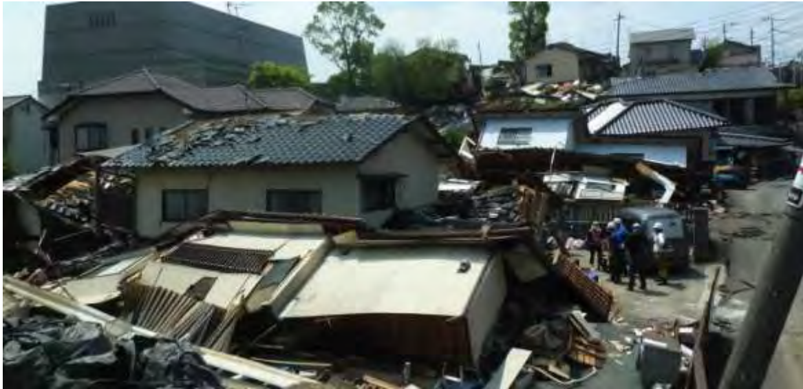
Another view of a heavily damaged residential area of Mashiki. All of the houses in the photo are wood frame; most are relatively new.
