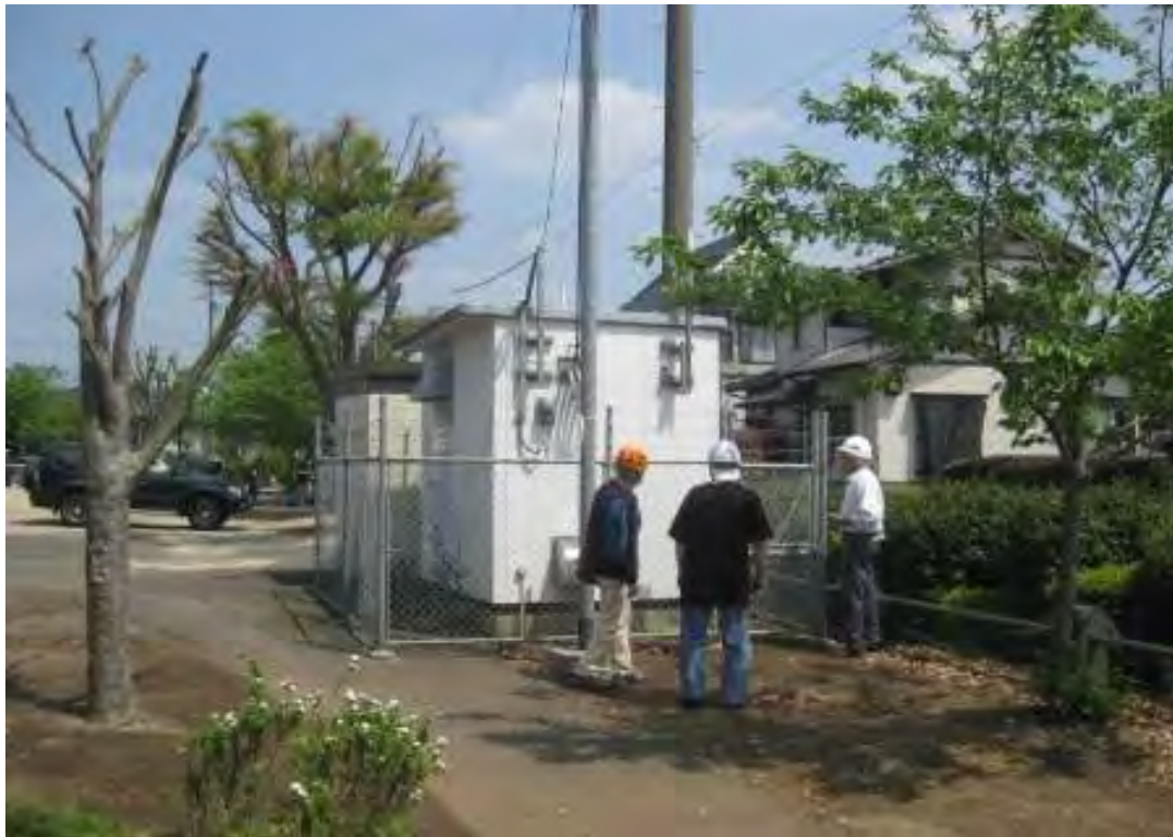
The strong motion instrument nearest the area of heavy damage is located in a small concrete shed in a park atop the ridge bounding the north side of Mashiki Valley. The instrument recorded a peak of 1.18g in the east-west direction, averaging 0.93g horizontal.
