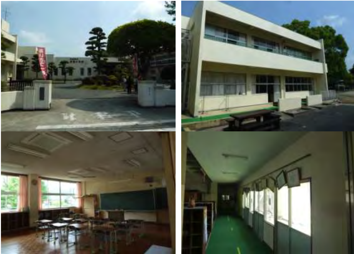
Additional photos of the practically undamaged interior and exterior of the elementary school.
