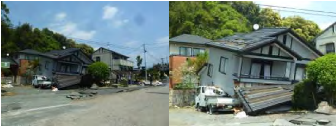
Another house with too many openings (windows) and not enough walls on the ground floor. Note the relatively undamaged houses behind and on the right of the collapsed house.
