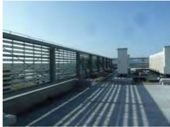
partial view of one of the two story hospital buildings (left) and the undamaged steel framed and braced parapet on the roof of the 6-story main building.
