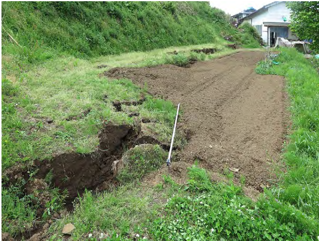
Figure 2 Surface rupture at Shimojin (N32.49519° E 130.84871°)
