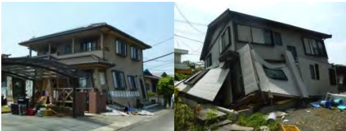
Another house with too many openings (windows) and not enough walls on the ground floor. Note the relatively undamaged houses behind and on the right of the collapsed house.
