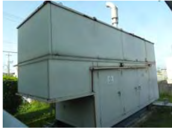
Other anchored equipment at ground level had no damage, including the two potable water tanks on the left and a diesel generator on the right.
