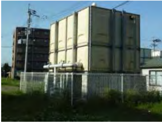
Other anchored equipment at ground level had no damage, including the two potable water tanks on the left and a diesel generator on the right.
