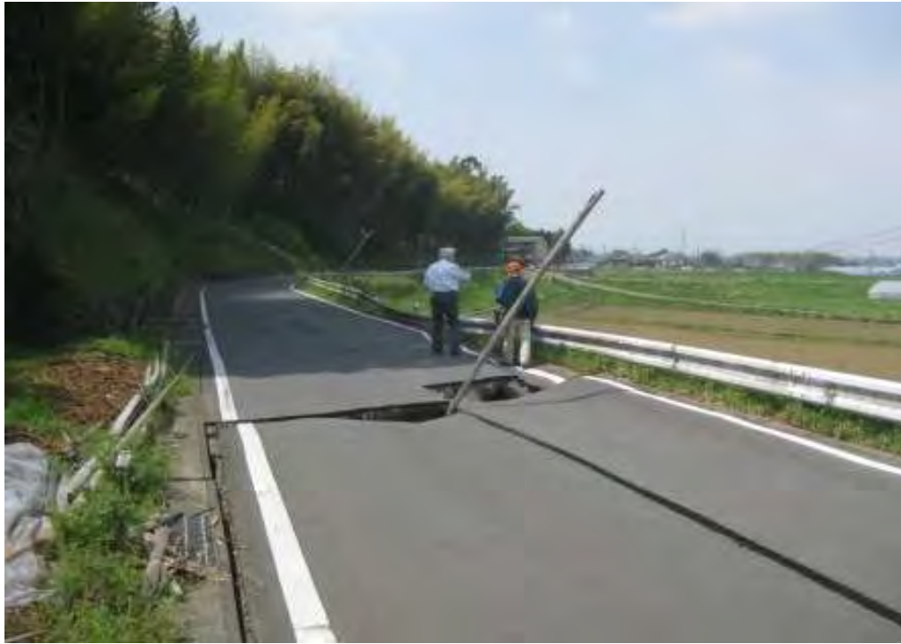
The surface trace of the fault on the southern side of the Mashiki Valley created offsets in roadways and retaining walls and in a few homes. The photo looks west along the Futogawa fault toward Kumamoto.
