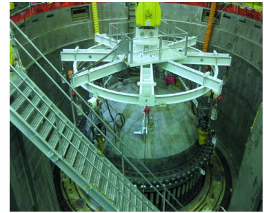
RPV Head Stud Tensioner Carousel
